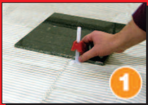
1 Insert straps under tile during installation.
